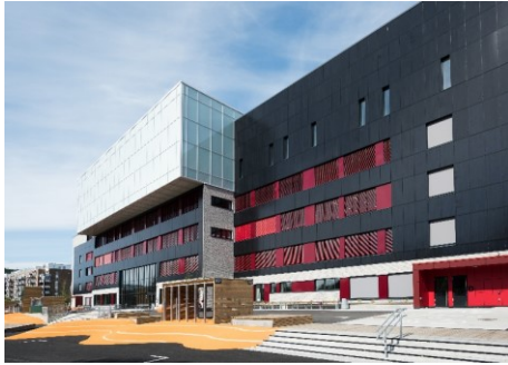
Brynseng skole – installert i fasade 163 kW peak
