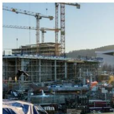
Zero-Emission Construction Sites
